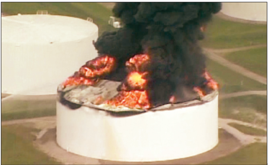
Obstructions caused this fire to behave like several fires in one tank
