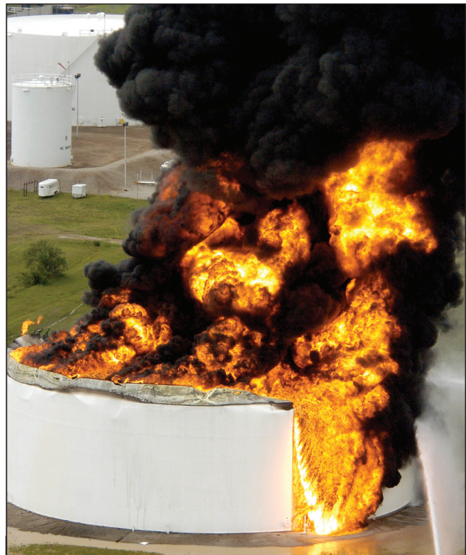
A wave sent through the product by the sinking pan gave the false impression of a tank wall failure.
