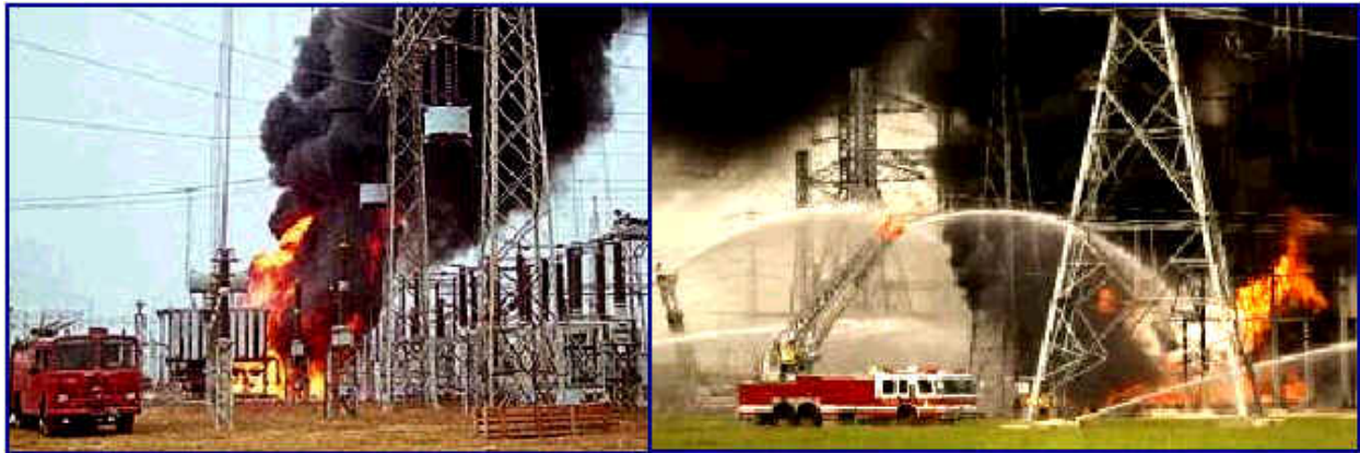
India, December 24, 2002, Ponchkula, Substation Ramgarh-Madanpur
